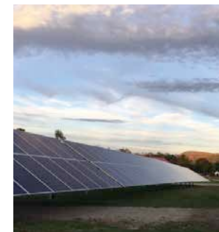
The solar array is located near the edge of the athletic fields on the south end of the campus.
